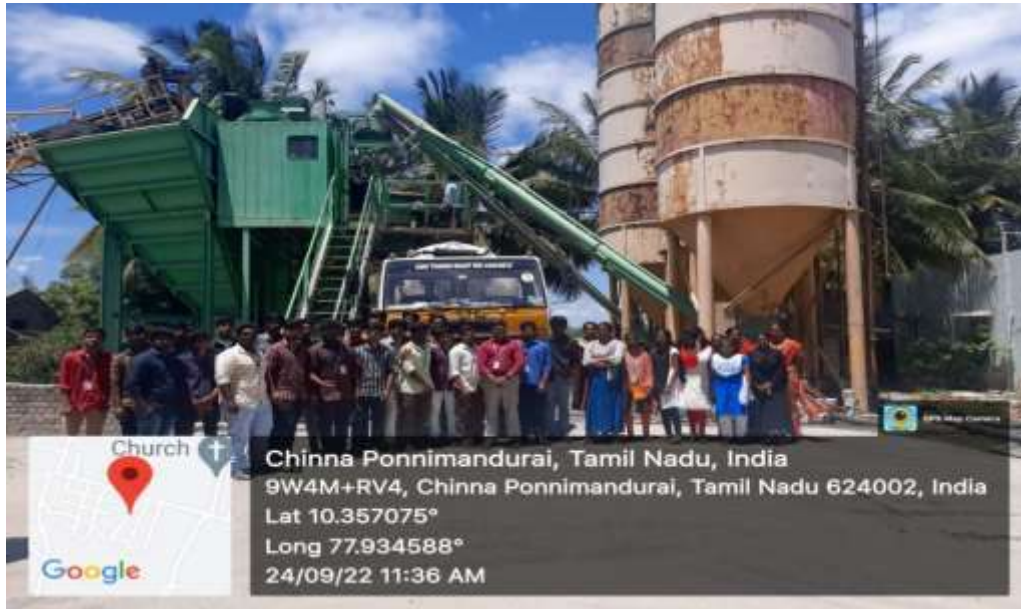
Sri Dharani Ready Mix Concrete Plant, Dindigul
